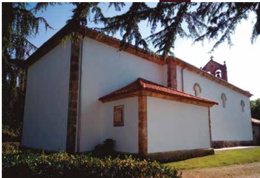
BEFORE - AFTER Ferroluz Universal Emulsion Façade Rehabilitation
